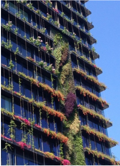
Integrated into the walls
