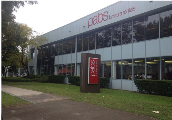
Figure 5.105: An example of a landscaped setback that presents well to the street and softens the appearance of the building
